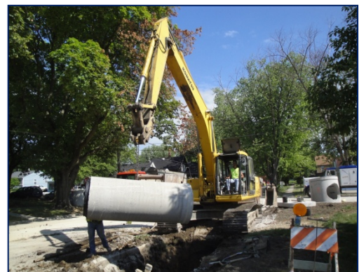
Figure 7. Typical Storm Sewer Construction
