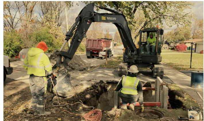
Completed in 2021, Phase I of SWM and DuPage DOT's **Kearney Road Dam Outlet Pipe Rehabilitation Project** involves replacing a culvert and slip lining 300 feet of storm sewer that conveys Wards Creek in unincorporated Downers Grove.
