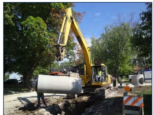
Figure 7. Typical Storm Sewer Construction
