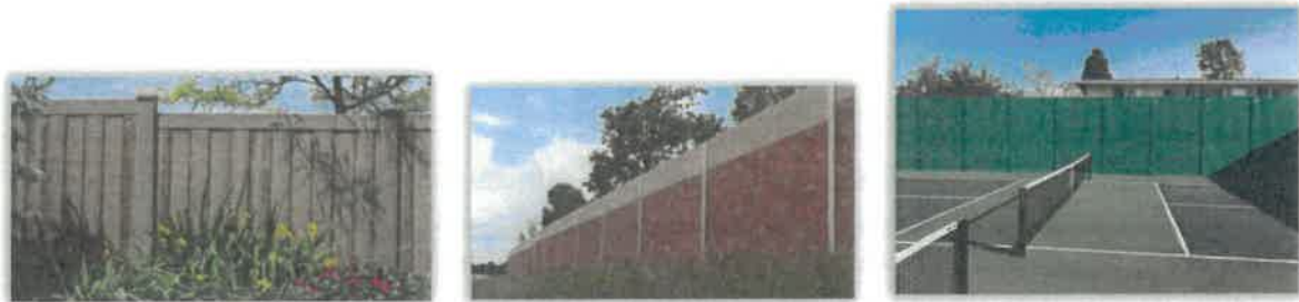
Figure 7 – Noise Wall Examples: SimTek wood look, concrete wall, and Acoustifence
