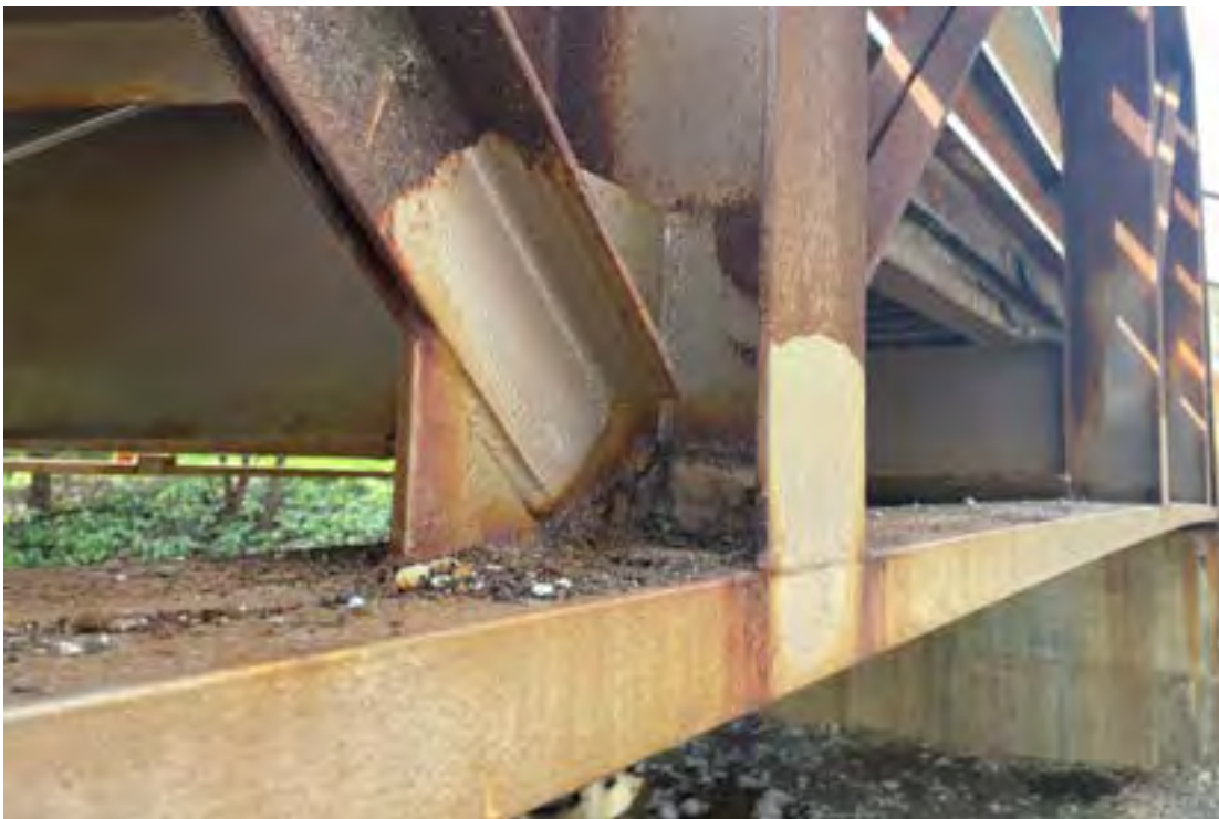
Gusset Plate Welded Connections of Truss Members at Midspan (East Side, Bottom Chord looking North)
