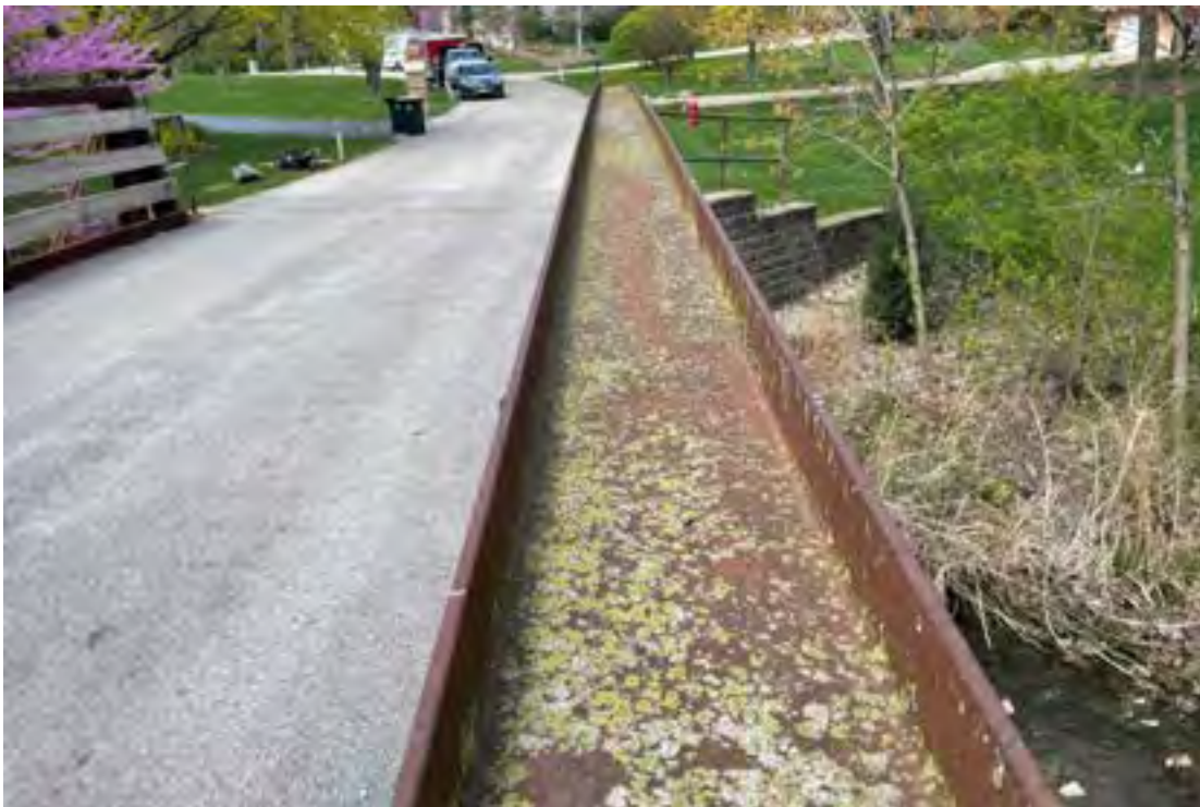
Top of Top Chord – Minor Surface Rust/Pitting
