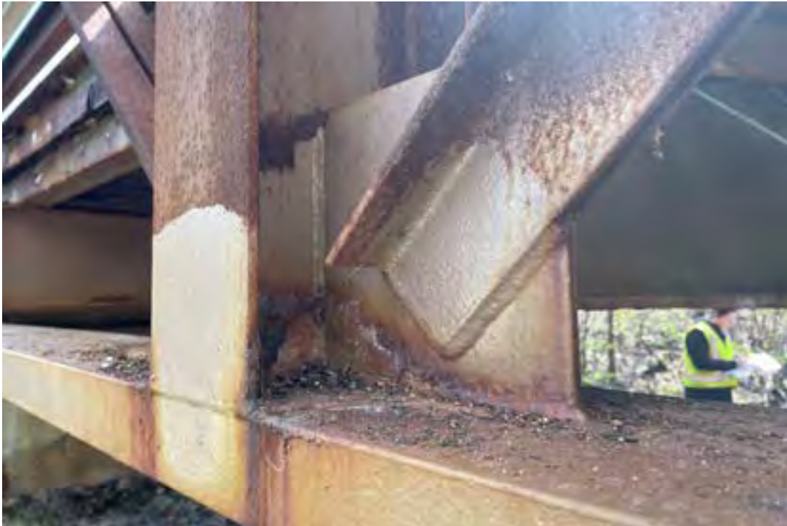
Gusset Plate Welded Connections of Truss Members at Midspan (East Side, Bottom Chord looking South)
