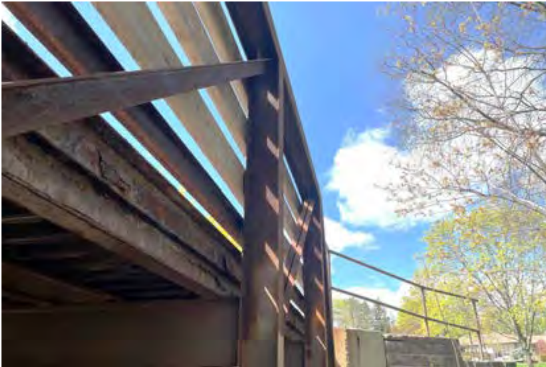
Typical Vertical Member of Truss (East Side, North of Center Shown)
