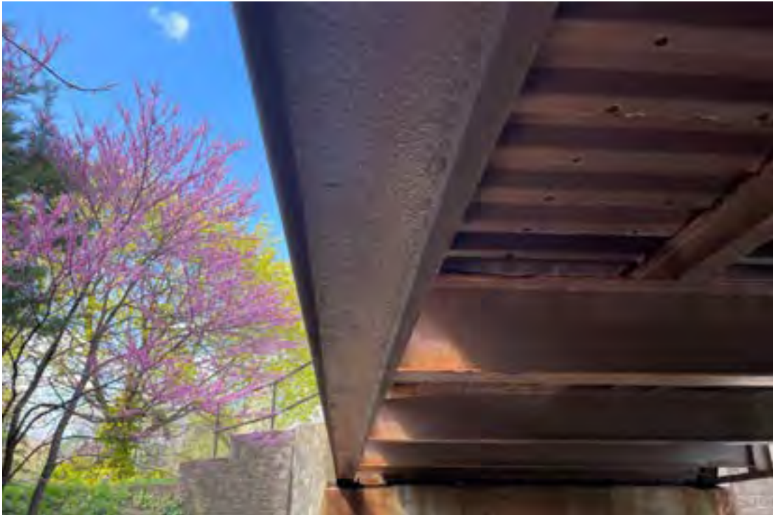
Bottom of Bottom Truss Chord, West Side – Initial Section Loss
