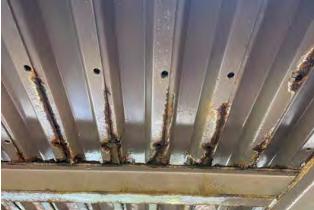
Deck Pan (East side, North of Center), Complete Section Loss Adjacent to Stringer 15" W x 3'-3" L - Recommend Repair
