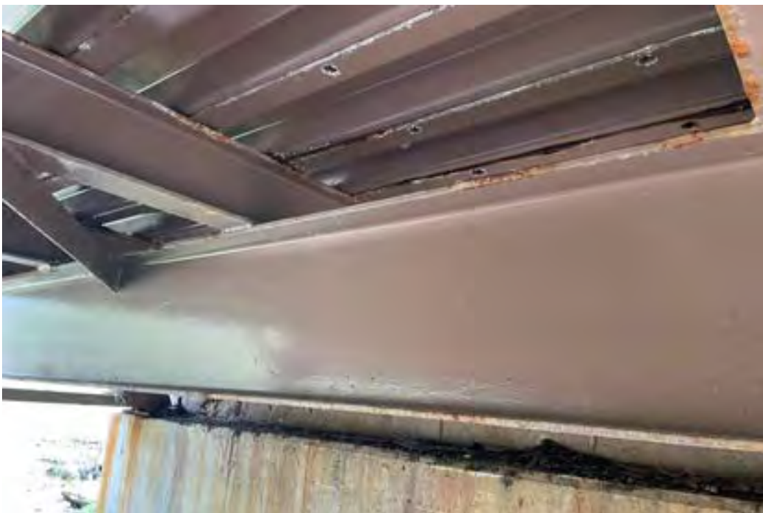
Typical Floor Beams (South End) – Initial Section Loss
