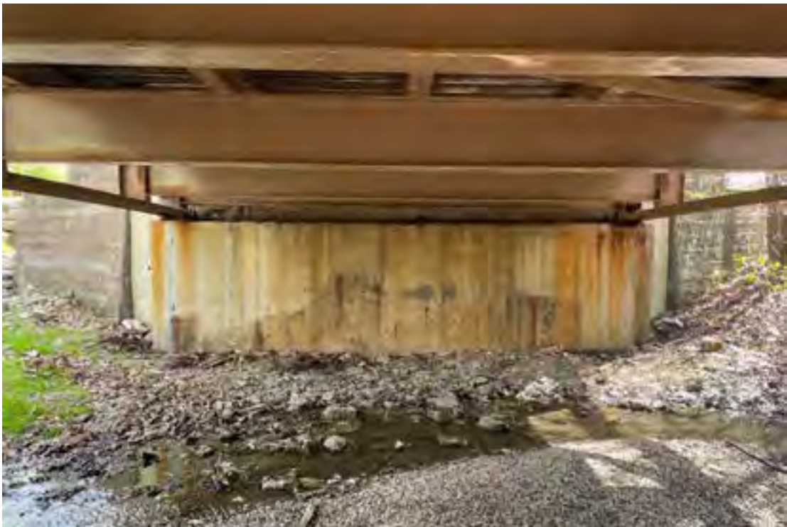
South Abutment – New Spall in East side of Backwall
