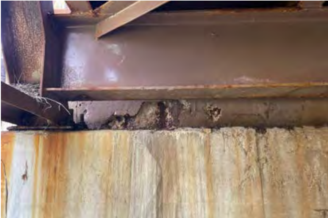
Close-up of 2' x 2' Spall in Backwall of South Abutment, East Side
