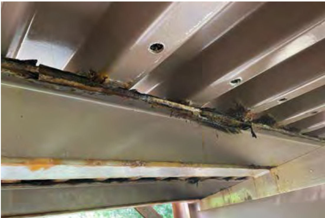
Typical Stringer (South End), Rust and Section Loss in Top Flange
