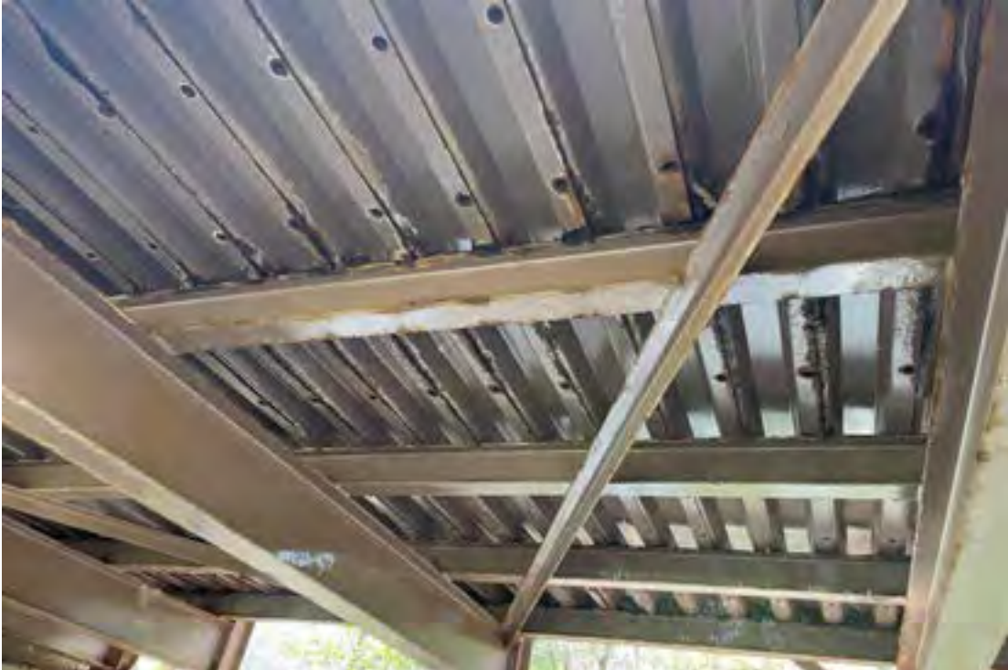
Typical Underside of Bridge (Midspan) – Initial Section Loss at Several Locations in Deck Pan, Floor Beams and Stringers, Painted in 2018 – Paint is Failing in Several Locations
