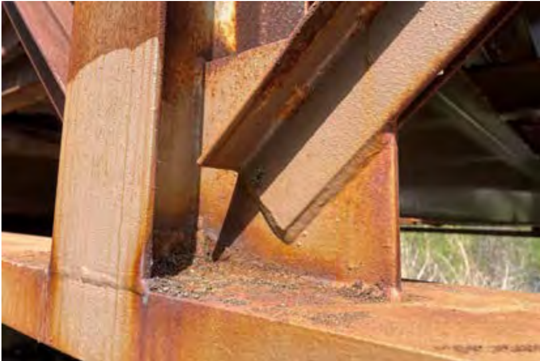
Gusset Plate Welded Connections of Truss Members at Midspan (West Side, Bottom Chord)
