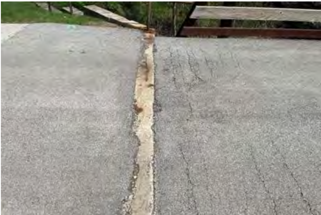
North Bridge Joint looking East –Minor Deterioration/Spalling of Backwall
