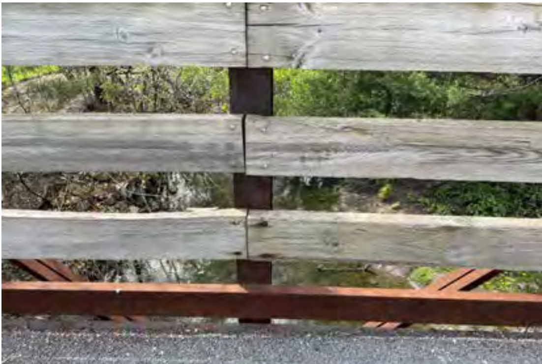
Bottom Rail of West Railing – Repaired since Last Inspection
