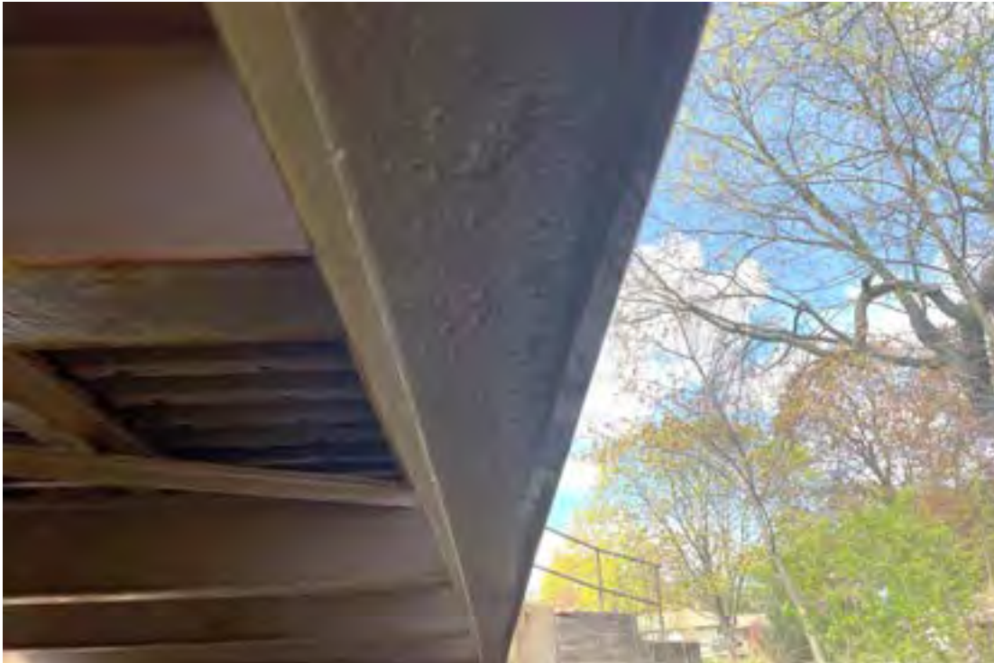
Bottom of Bottom Truss Chord, East Side – Initial Section Loss
