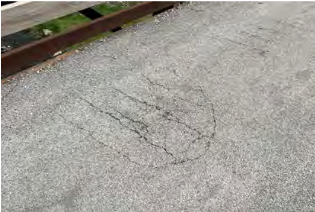
Pavement Cracking and Settling above Deck Pan with Section Loss – Midspan, East Side
