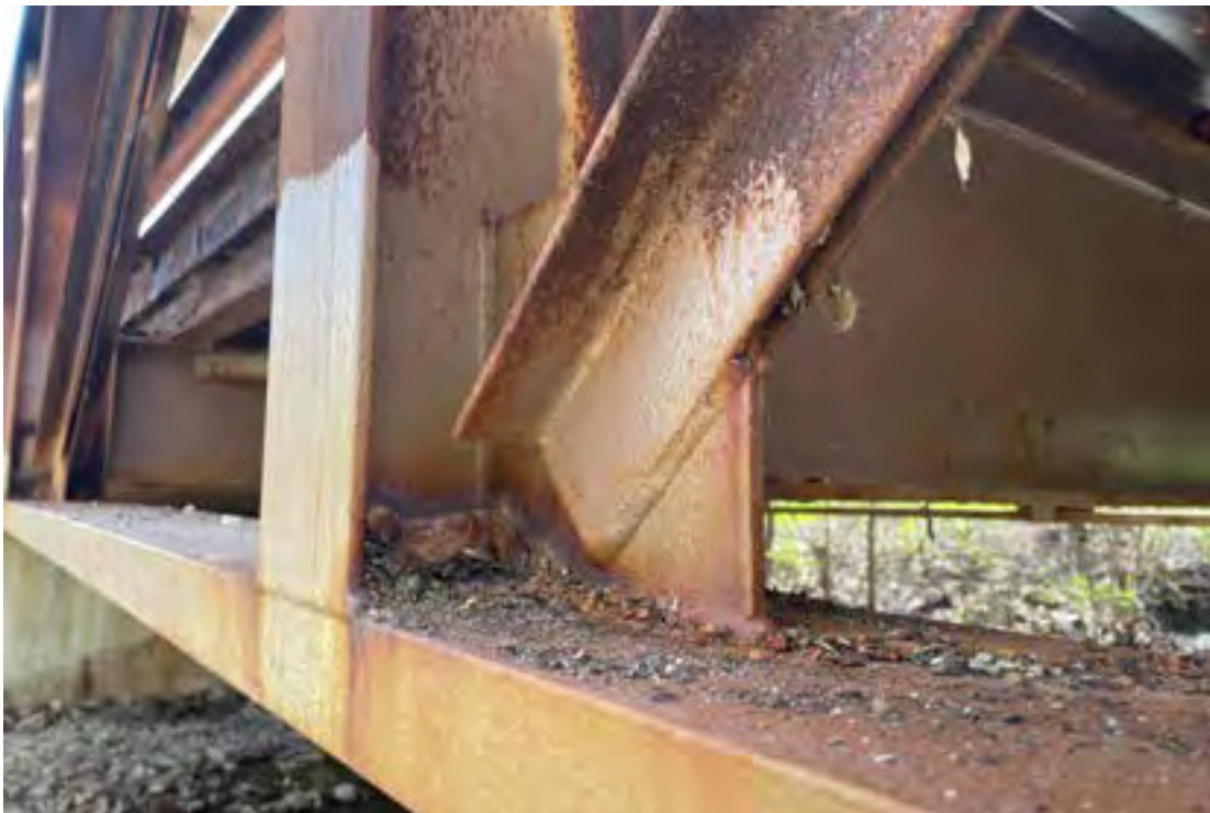
Gusset Plate Welded Connections of Truss Members at 1/4 Span
