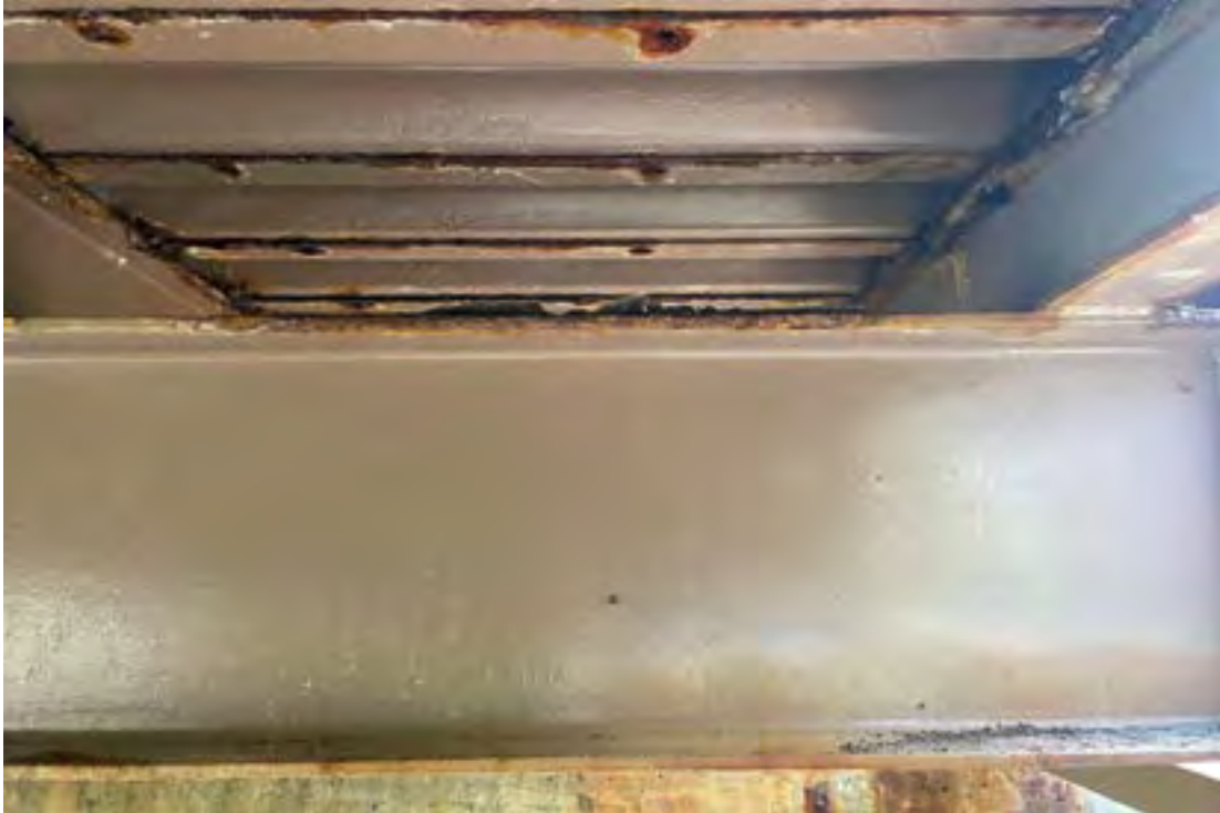
Rust and Section Loss in Top Flange of Floor Beam (Typical)
