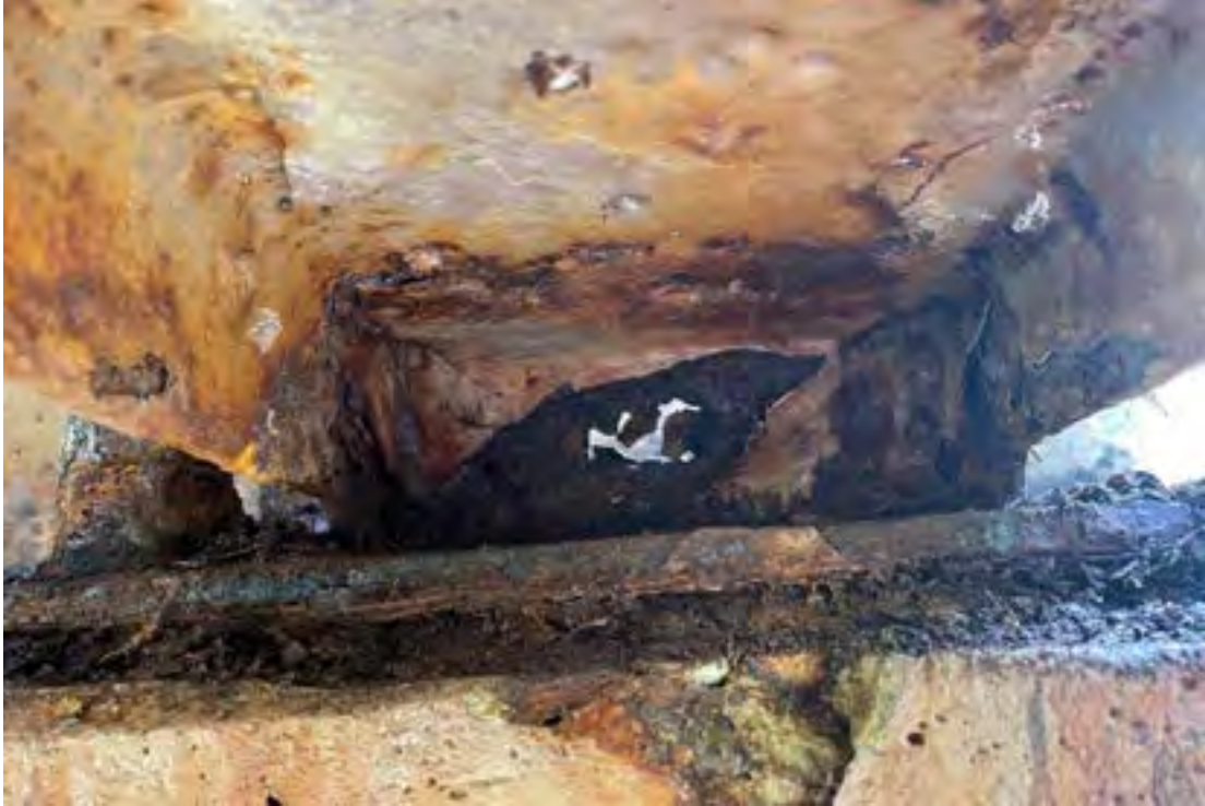
Southwest Truss Bearing – 1" H x 1 3/4" W Hole in Web of Diagonal under Bottom Chord – Consider Repair
