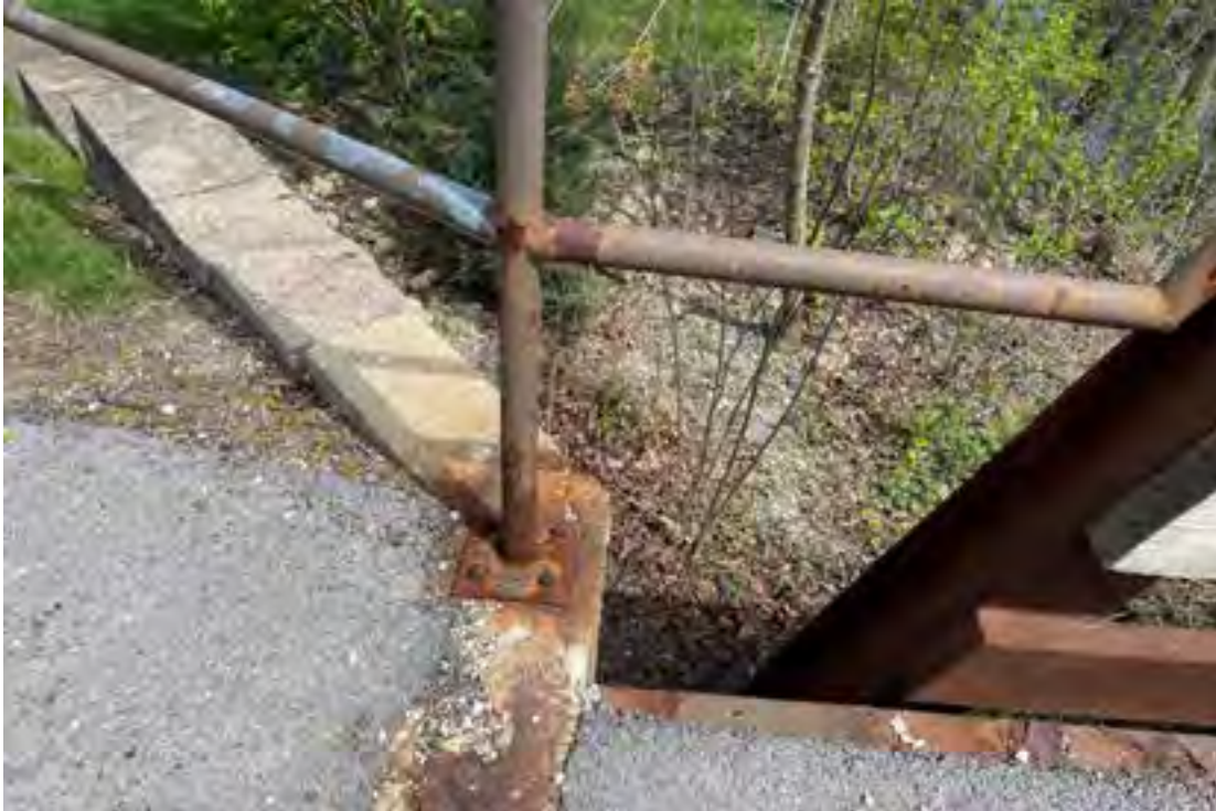
Handrail Attached to Wingwall – Moderate Corrosion at Base
