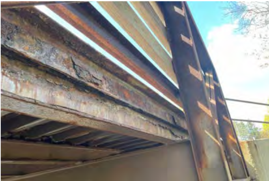
Exterior Stringer and Side Strut – Paint Failing, Pack Rust and Section Loss along Exterior Stringers(Typical)
