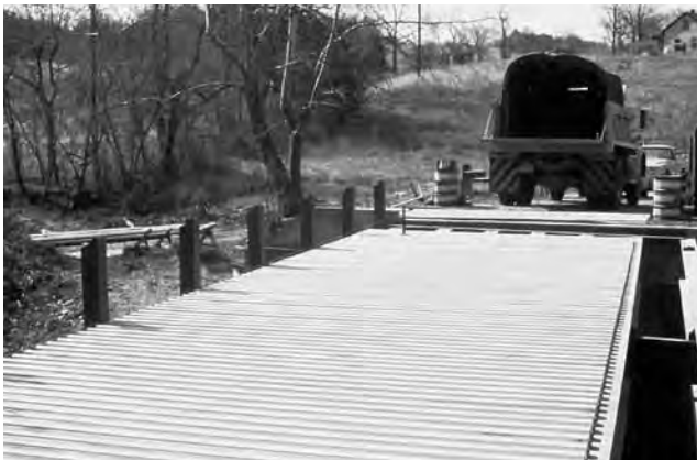
Bridge planks are easily bolted or welded into place to form a continuous bridge deck.
