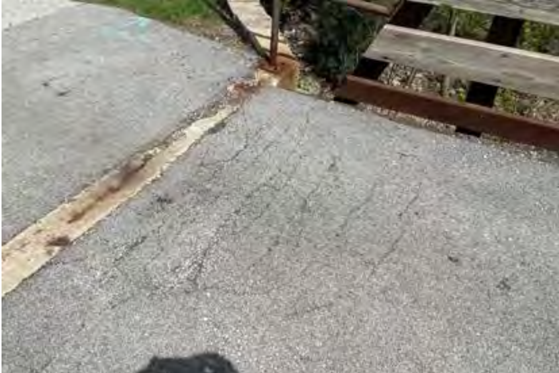
Pavement Cracking and Settling above Deck Pan with Section Loss – Northeast Corner
