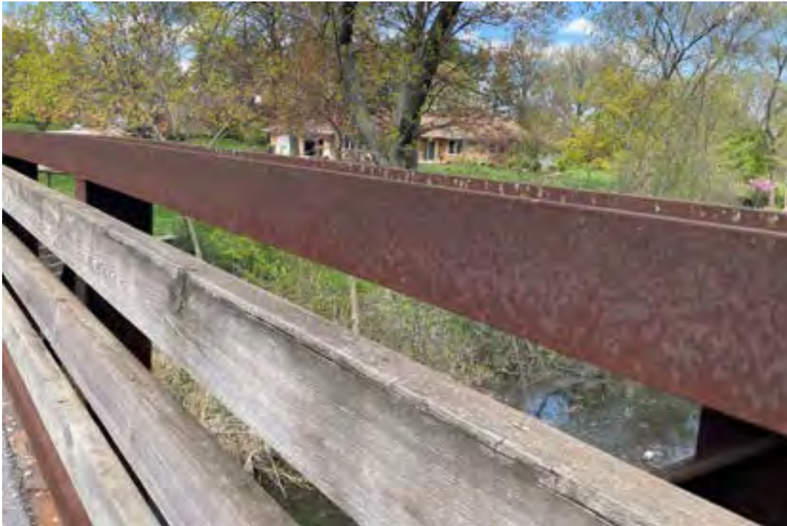
Steel Superstructure Elements (Top Chord Shown) – Minor Surface Rust/Pitting
