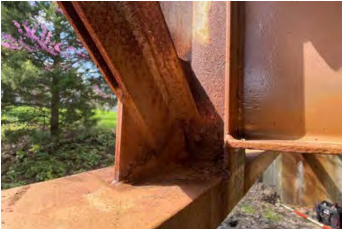
Substructure Gusset Plate Connection @ Midspan – West Side
