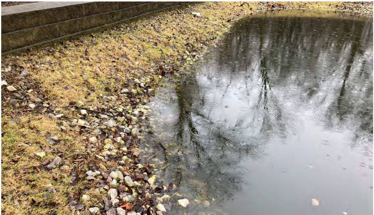
Photo 4. Rocks used as stabilization along excavated pond banks. Facing southwest.
