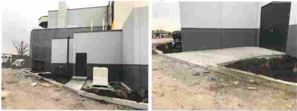
Exhibit 2 Addition of ADA ramps and fire connection
