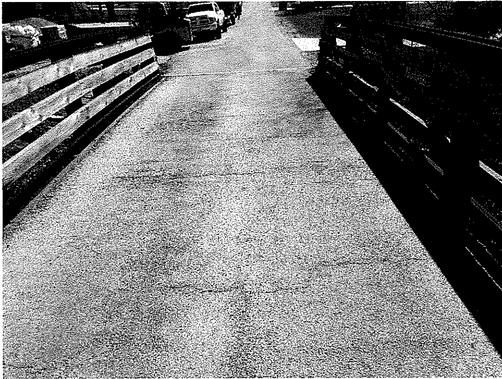
HMA Deck Condition – Cracking Noted Throughout
