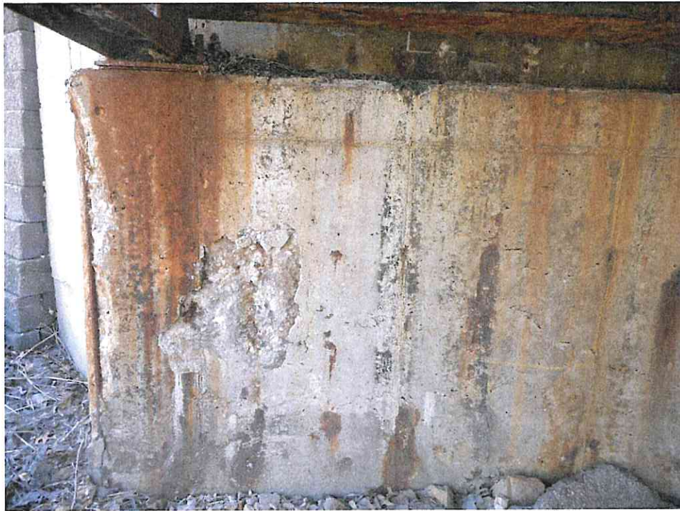
South Abutment – Delaminations and Spalling with Exposed Reinforcement
