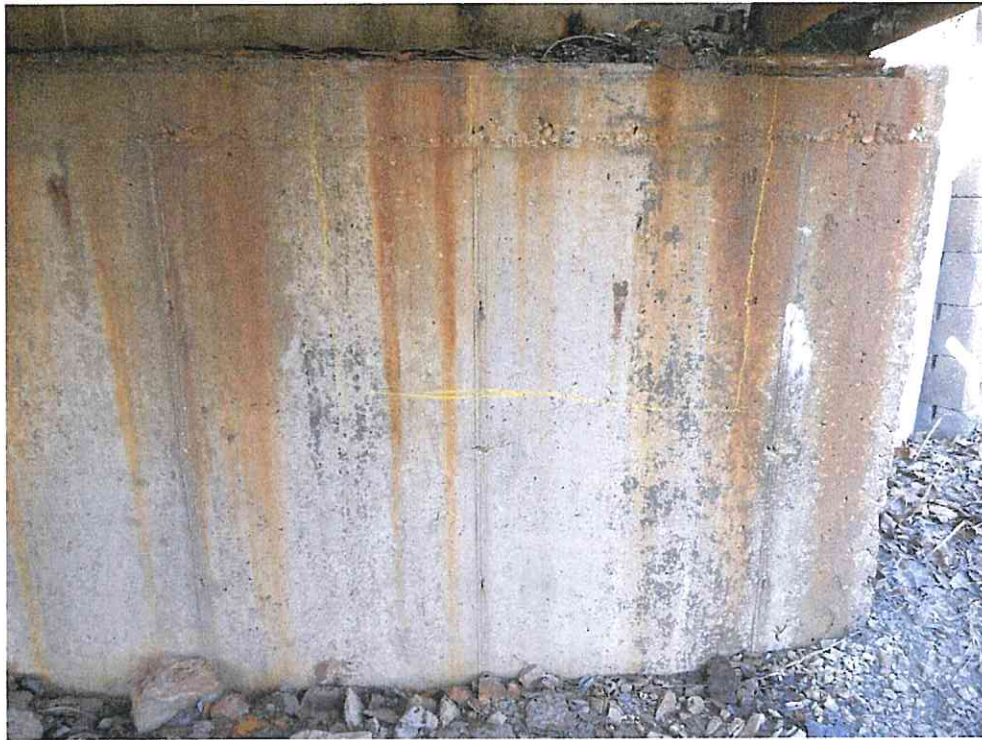
North Abutment – Delaminations Noted
