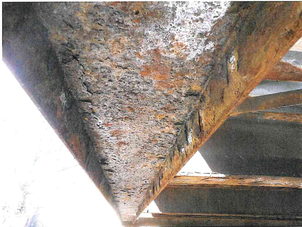
Pack Rust on Underside of Truss Bottom Chord
