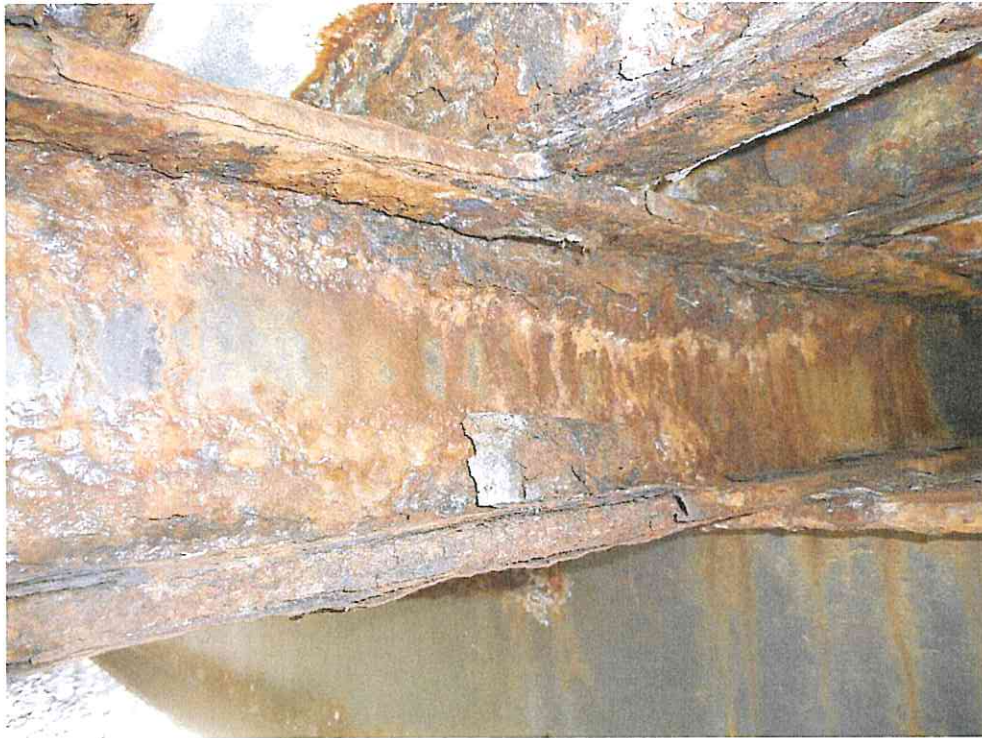
Underside of Bridge – Pack Rust on Metal Pan and Stringers
