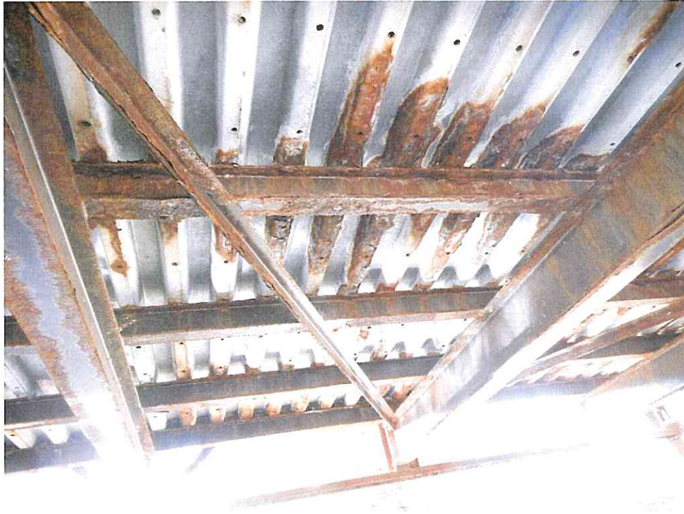
Underside of Bridge – Pack Rust on Metal Pan, Floor Beams, Stringers and Diagonal Bracing
