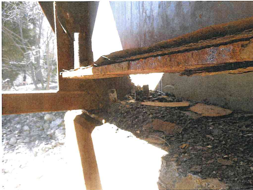
Underside of Bridge – Pack Rust on Floor Beam
