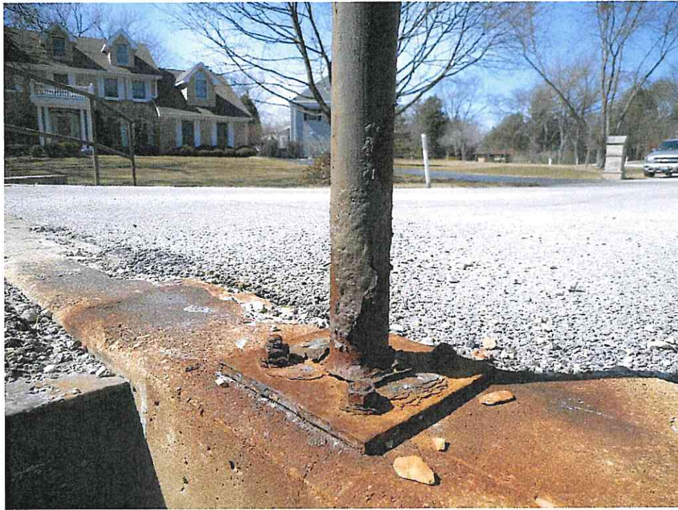
Railing – Post Corrosion
