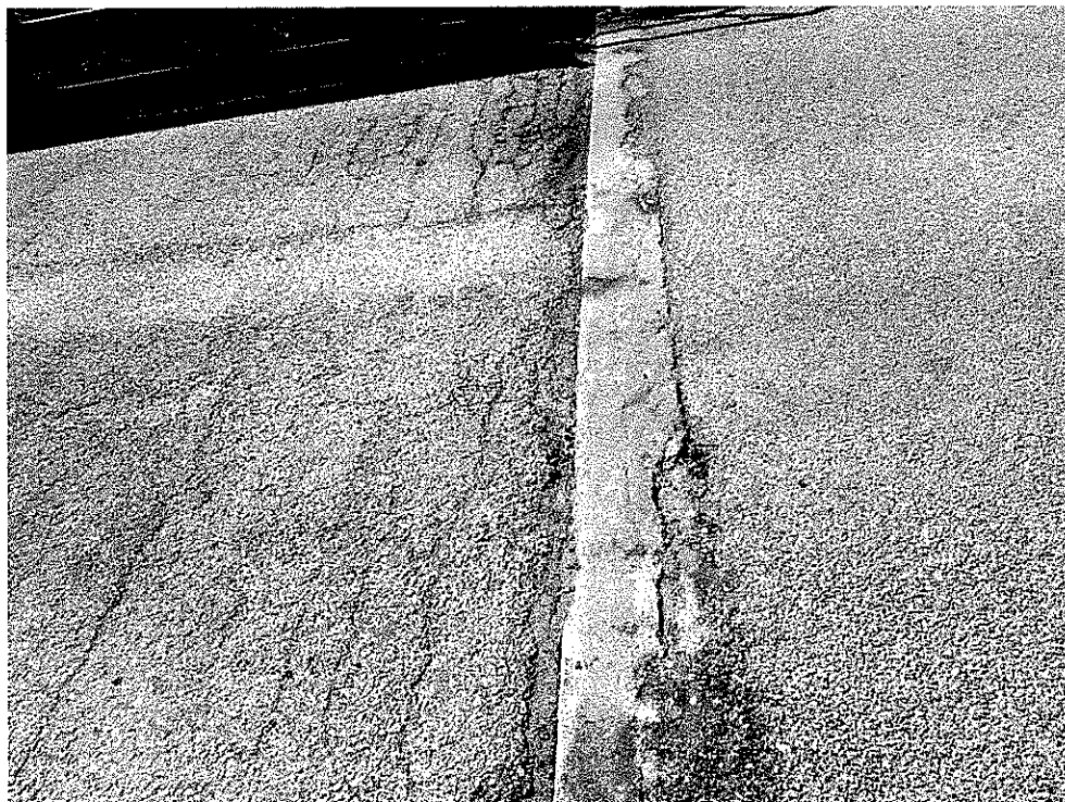
North End of Bridge – Backwall Cracking and Spalling – Joint Filled with HMA/Debris
