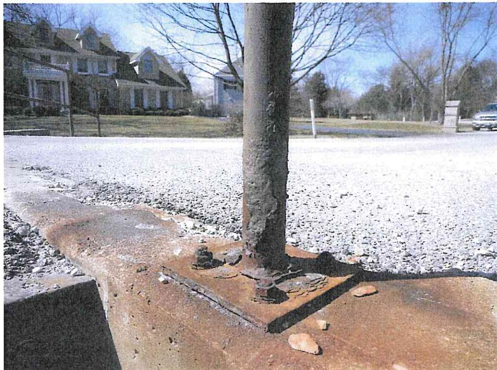
Railing – Post Corrosion
