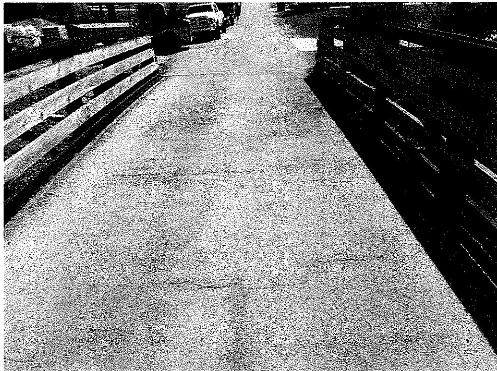
HMA Deck Condition – Cracking Noted Throughout
