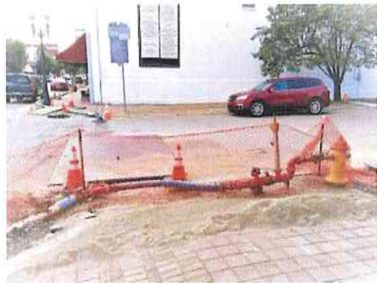
The bypass system for the Huntingburg, Indiana relining project.
