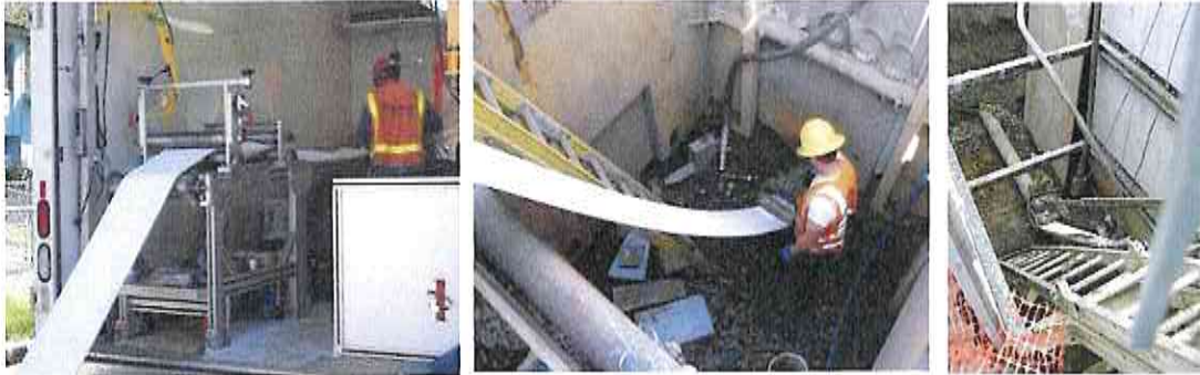
Figure 16: Insertion of the liner
