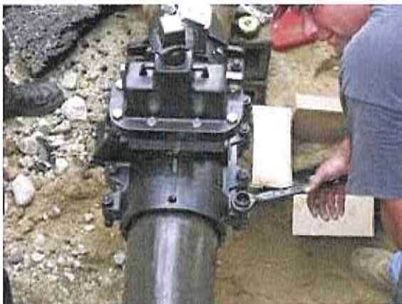
Figure 24: Typical Pipe Cut
