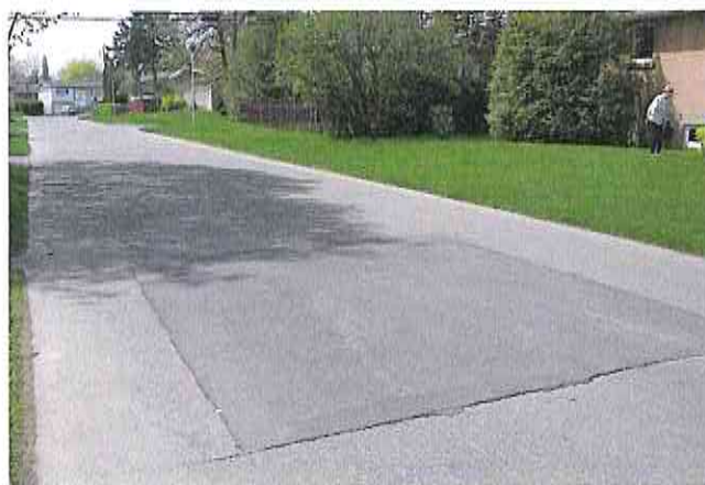
Figure 4: Paving after CIPP rehabilitation
