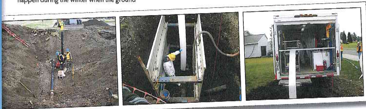
Replacing pipes using traditional (non-trenchless) methods requires 40-wide excavation (left). During pipe repair at JBER using trenchless technology, a flexible liner is impregnated with epoxy (right), then pulled into existing pipe (center). (U.S. Air Force photos)
