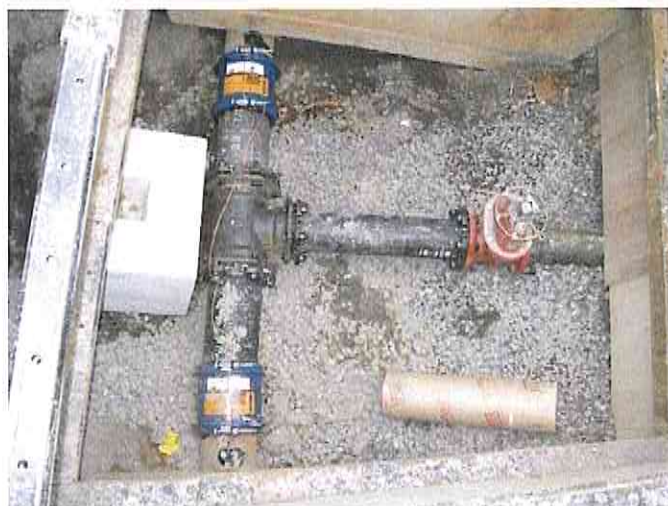
Figure 22: Typical Reconnection in an Insertion Pit
