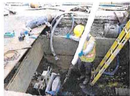
A Fer-Pal USA worker installs the AquaPipe liner in Huntingburg, Indiana.
