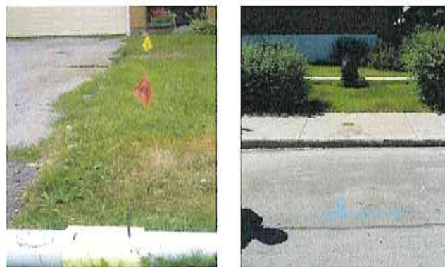
Figure 1: Locating the pipe
