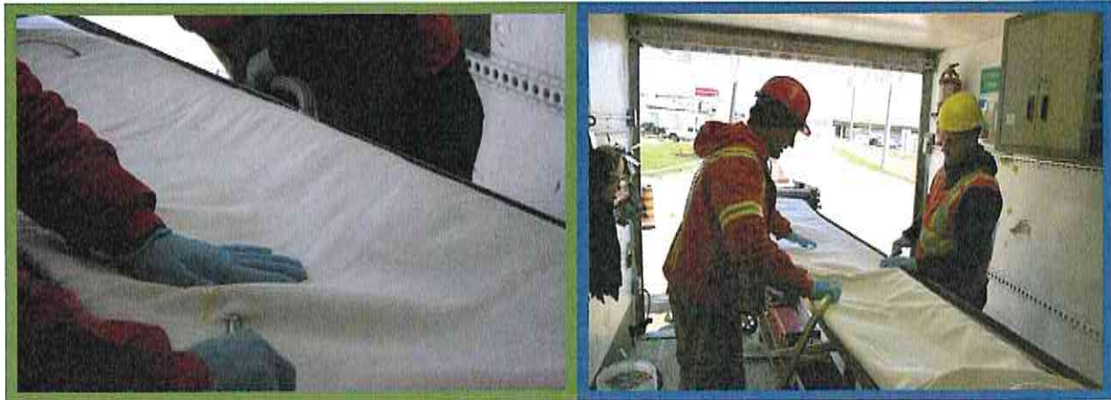
Figure 14: Impregnation of the jacket
