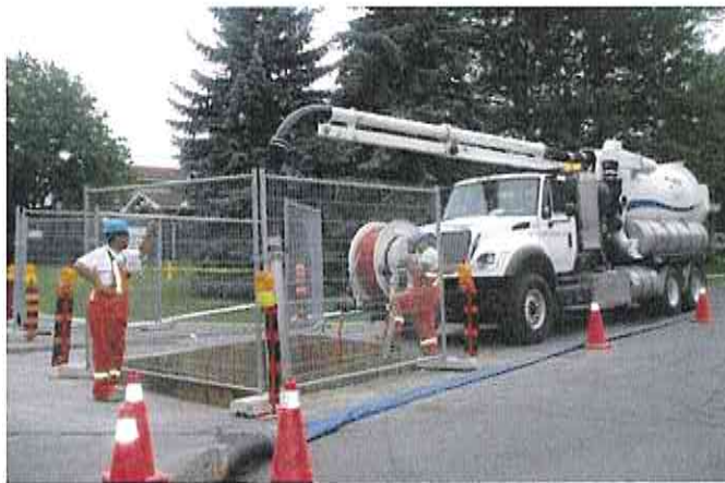
Figure 6: Trench Box and Fencing
