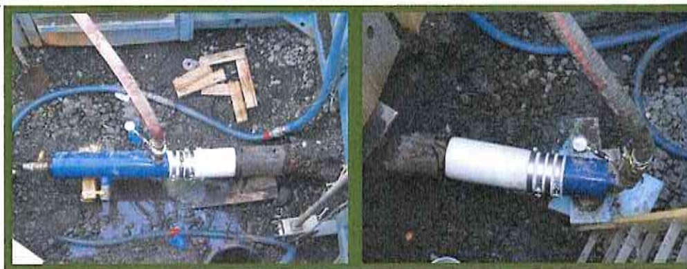
Figure 18: Curing with hot water
