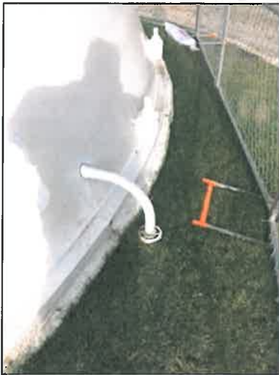
EXISTING CONDUIT PENETRATION ON EAST SIDE OF THE BASE CONE, CONTINUES AROUND THE INTERIOR PERIMETER OF THE TANK AND ENTERS THE NORTH SIDE OF THE CONTROL ROOM
