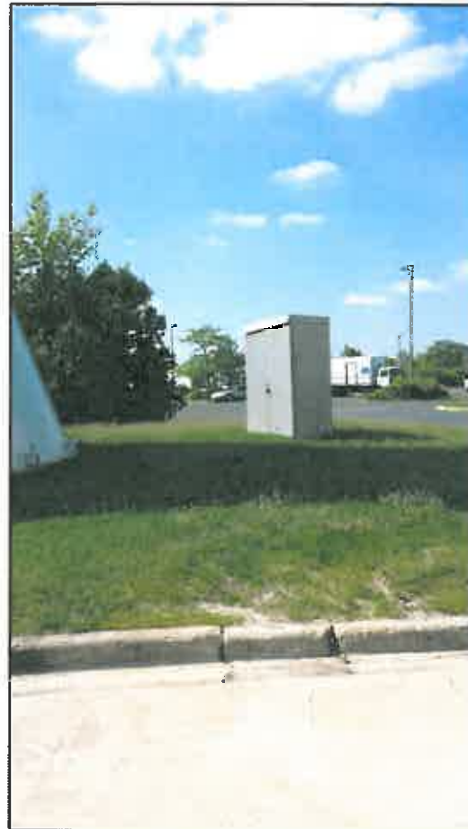
EXISTING TELEMETRY AND POWER CABINET LOCATED APPROX. 10' WEST OF TANK. TELEMETRY CABINET SHALL BE PROTECTED DURING CONSTRUCTION.
