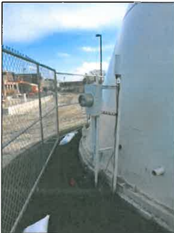
EXISTING COM ED METER AND SCADA ANTENNA MOUNTED ON UNISTRUT ON THE NORTH SIDE OF THE TANK. ALL EQUIPMENT SHALL BE PROTECTED DURING CONSTRUCTION.
