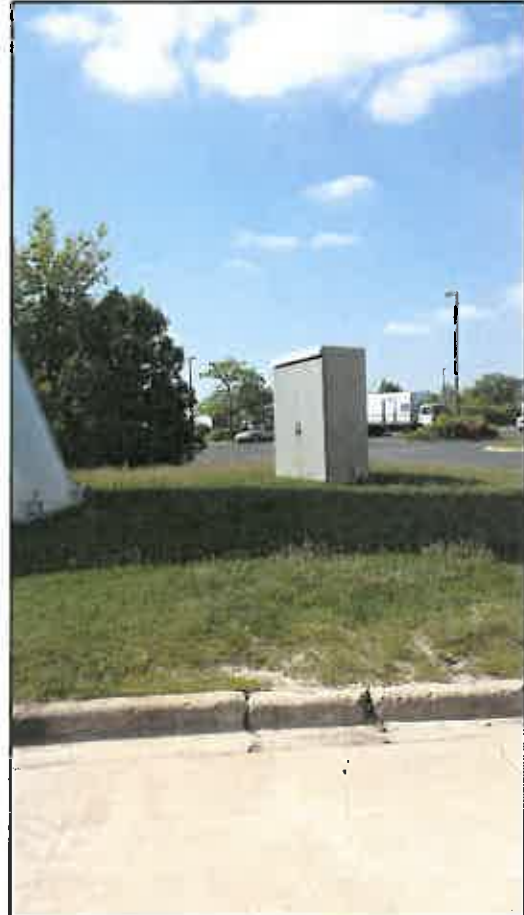
EXISTING TELEMTRY AND POWER CABINET LOCATED APPROX. 10' WEST OF TANK. TELEMTRY CABINET SHALL BE PROTECTED DURING CONSTRUCTION.
