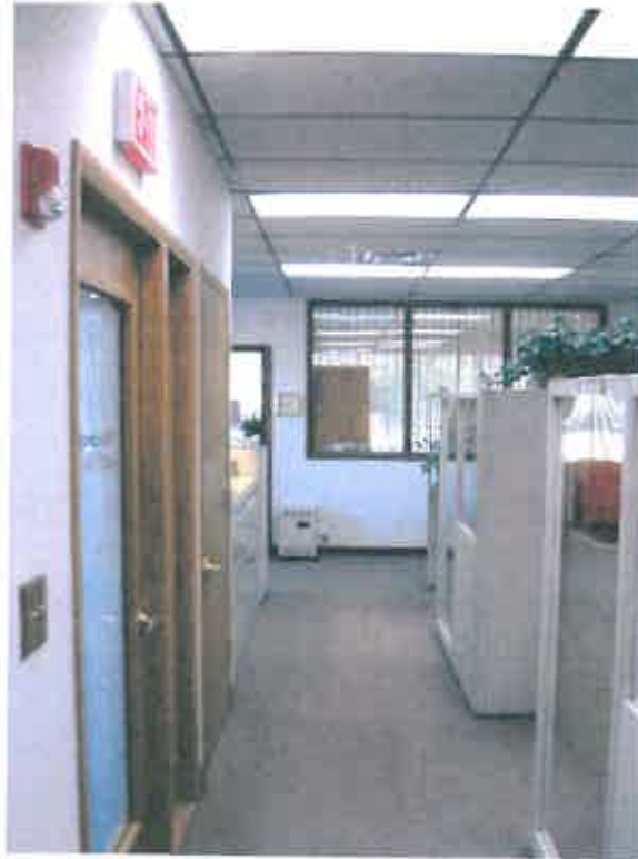
Figure 11 – Typical finishes of carpet, drywall and suspended ceiling tile in the tenant's offices.
