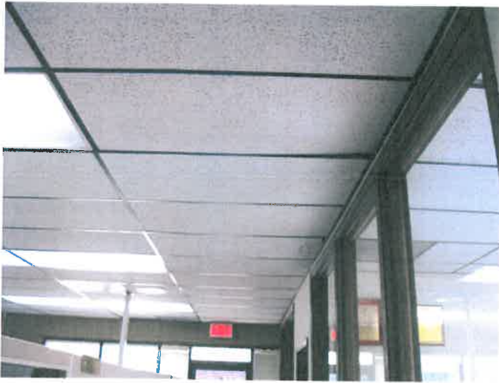
Figure 10 – Typical 2x4 ceiling tile and grid. Staining is apparent in several locations.
