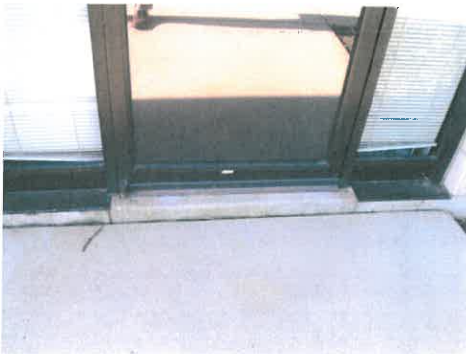
Figure 4 – Concrete walk at entrance door on north wall has settled.
