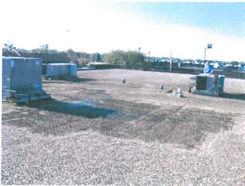
Figure 2 – Ballasted asphalt roof in poor condition.
