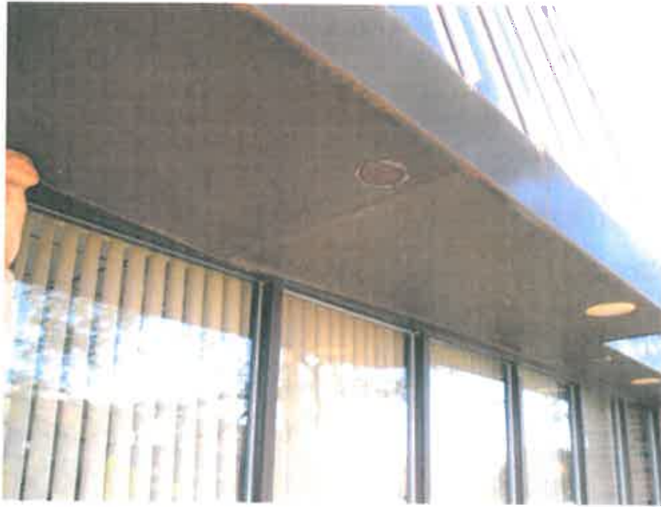
Figure 5 – Exterior soffit sagging on north wall.
