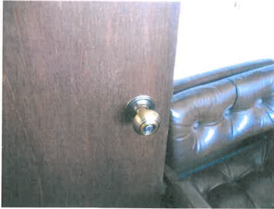
Figure 9 – Knob hardware on selected doors is not accessible.
